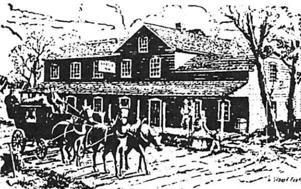
Still standing in Ogden av., Hinsdale, Castle Inn formed center of suburb's activity 120 years ago. Society plans annual publication treating historic places.
